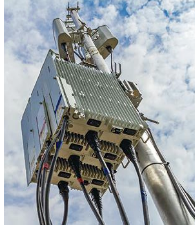
The entire market for telecommunications equipment is expected to surpass $500 billion between 2014 and 2019, according to the Dell'Oro report. (Image courtesy of ThinkStock).
